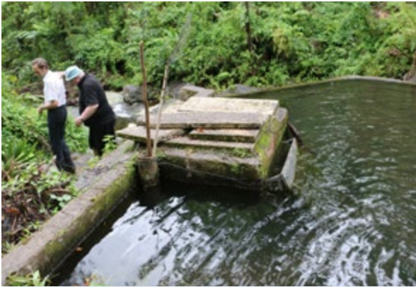
The dam at Tutu Rural Training Centre, Fiji.
