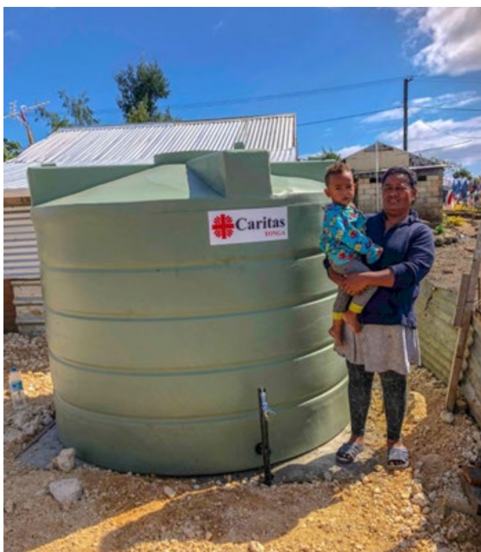
Fakei Latu and her baby next to a water tank installed outside her house. The tank serves 19 people around low lying Pa Tangata near Nuku'alofa, Tonga.
