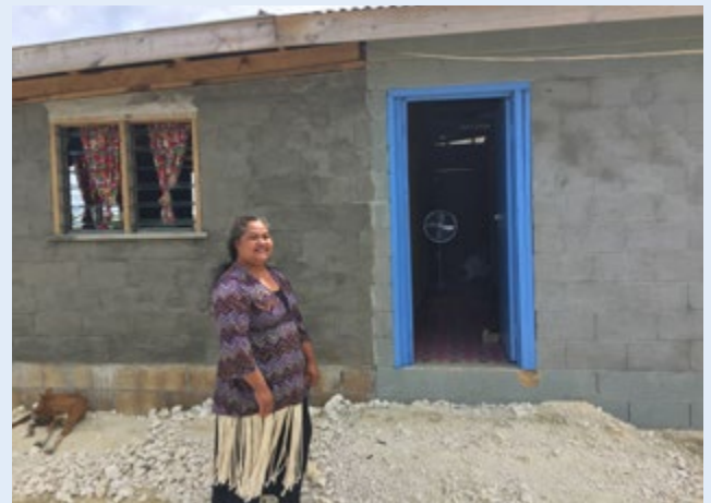
Katalina with newly completed house in 2016.
