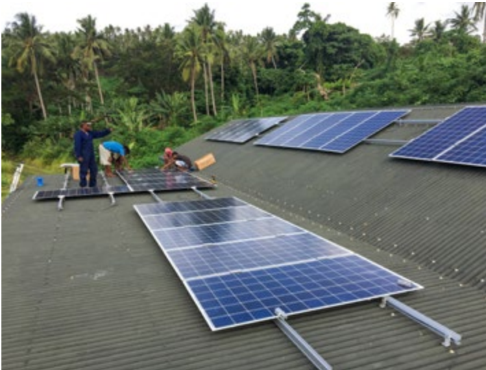
Installing solar at Tutu Rural Training Centre, Fiji.
